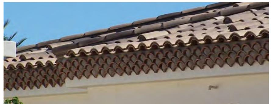
Stack booster tile 3 or 4 layers high under the eave on the wall of the building to create a decorative eave. From the bottom to the top row, the exposure is adjusted to become longer until the top row matches the exposure of the eave tile on the roof.
