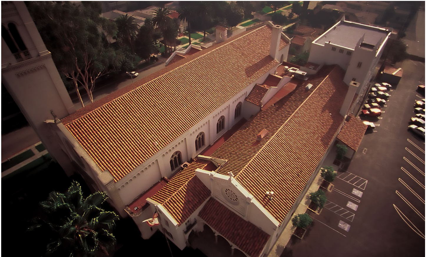
Wilshire United Methodist Church, Los Angeles, CA - 8" Straight Barrel Mission in custom colors to match original tile. The 1907 church interiors and roof were renovated in 1994 after unfortunate fires.
