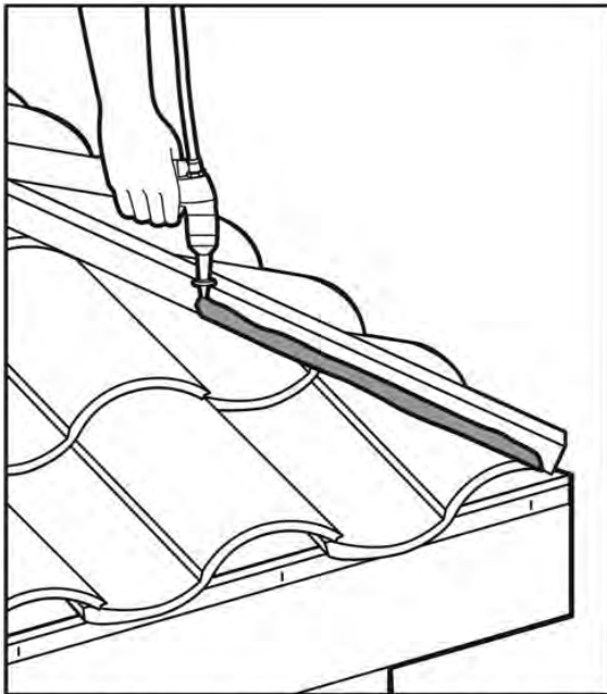
A bead of ICP Adhesives Polyset®AH-160 may be applied above the field tile surface on both sides of the hip/ridge board or galvanized frame
